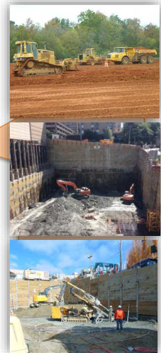
Pictures of sample rough grading, excavate, drill and grout tiebacks
