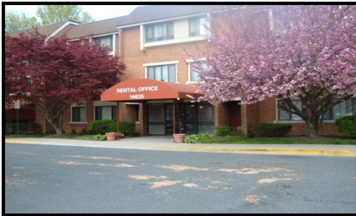
Current front entry taken from driveway off Bauer Drive, June 2018.
